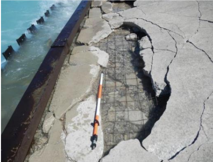
Interior Structure of Concrete Apron Visible
