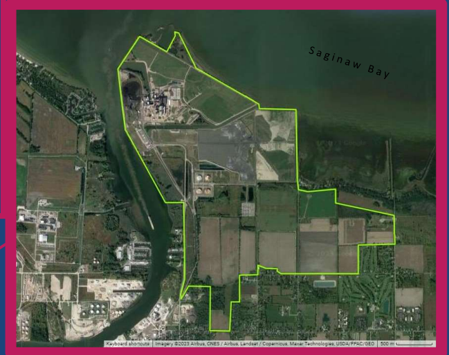
Dan E. Karn Power Plant Essexville, MI – Bay County Owned by: Consumers Energy
